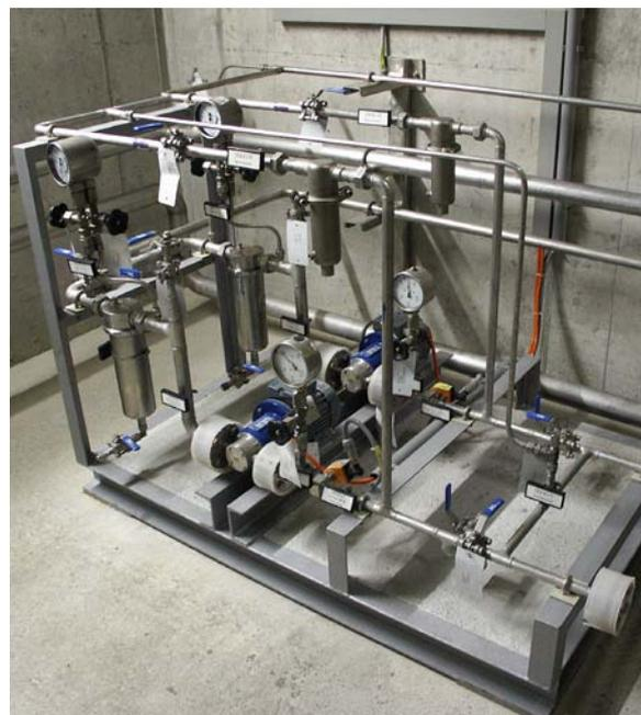
Fig. 2 Redundant pump station for additives
