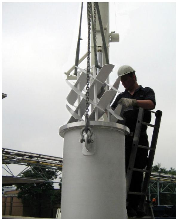
Fig. 1 Installation of static mixers in a tube reactor with a diameter DN800
