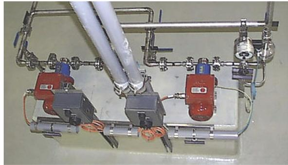
Fig. 5 KMD dosing modules integrated in the plant (installation and electrical work by Fluitec)
